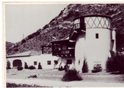
Laguna Beach Old Sewage Disposal Plant Exterior (to the left) and Interior (shown below.) The back of the interior photograph reads: "The sewage disposal plant at Lagoon, California, is architecturally unique. PWA funds financed the construction of this disposal plant." - National Archives and Records Administration
