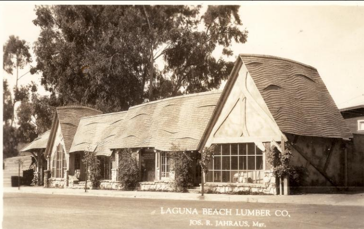
Laguna Beach Lumber Company Office Built in 1919 - Tom Pulley Postcard Collection
